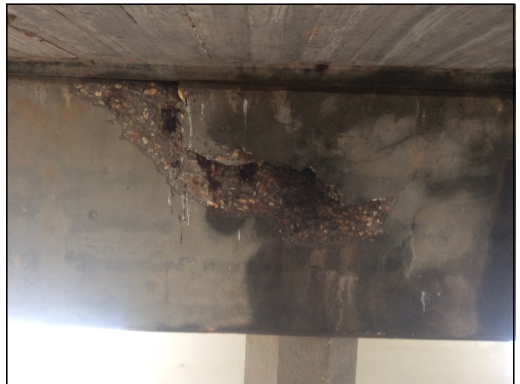
Crack Delams and spall with exposed rebar on bent 1 over pile 2&4
