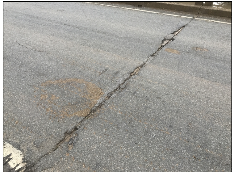
Joint - Bent 3: Deterioration of wearing surface (potholes)
