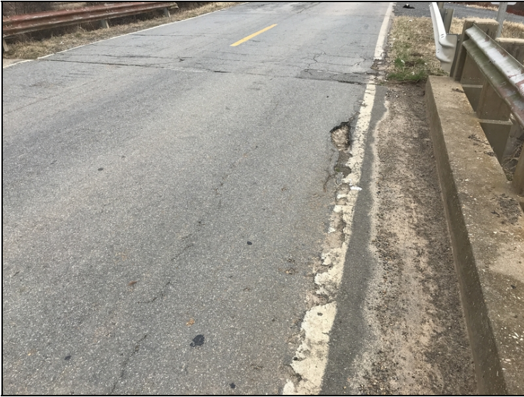
Wearing surface/deck - Span 4 right: Spalling
