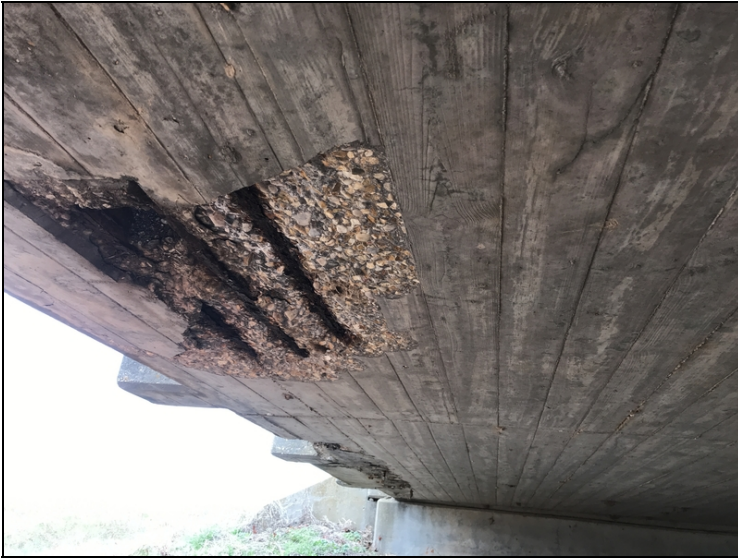
Soffit - Span 1 right: Rebar exposed
