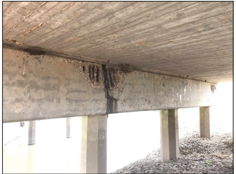
Cap - Bent 2 back: Rebar exposed
