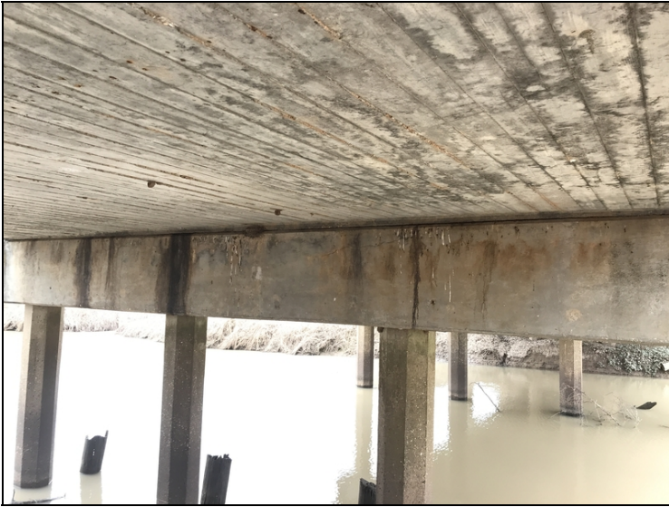
Cap - Bent 4 ahead: Cracking
