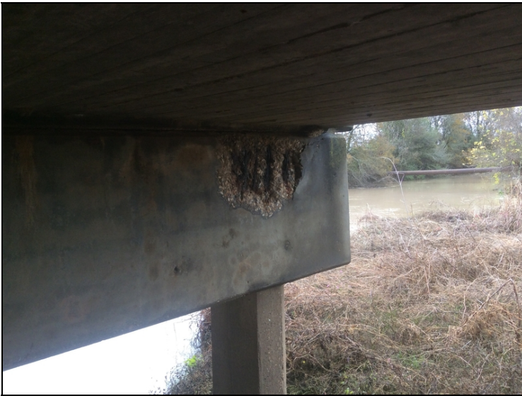
Spall with exposed rebar on bent 1 over pile 4
