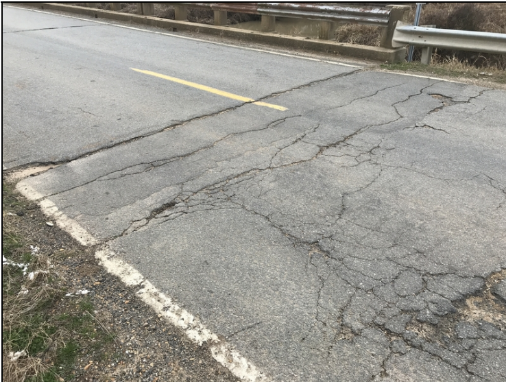
Approach roadway - Bent 1: Deterioration of wearing surface
